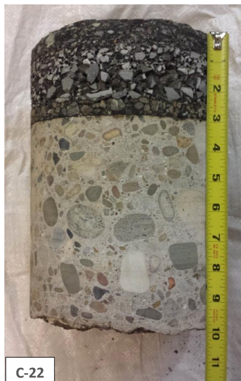
Figure 26-6 | Example of Pavement Core
