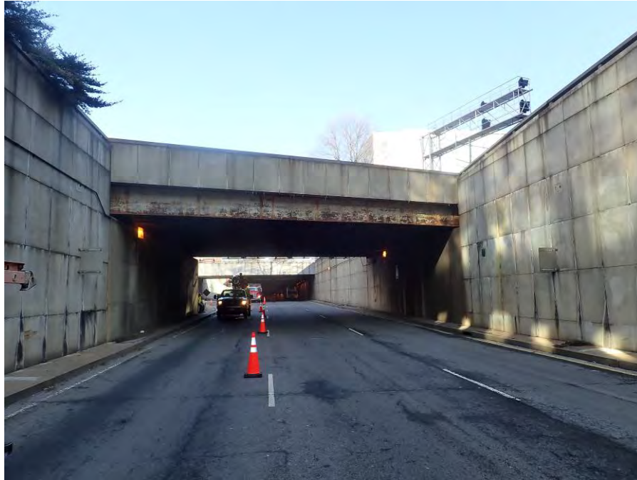
Photograph No. 1 – South Elevation, Looking North
