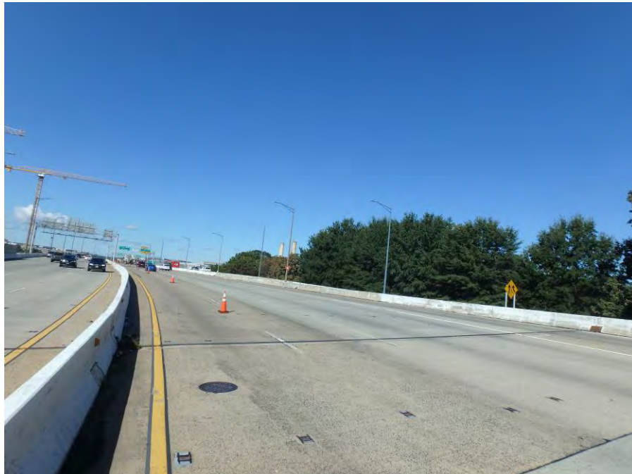
Photograph No. 8 – Westbound Lanes, East Approach, Looking West
