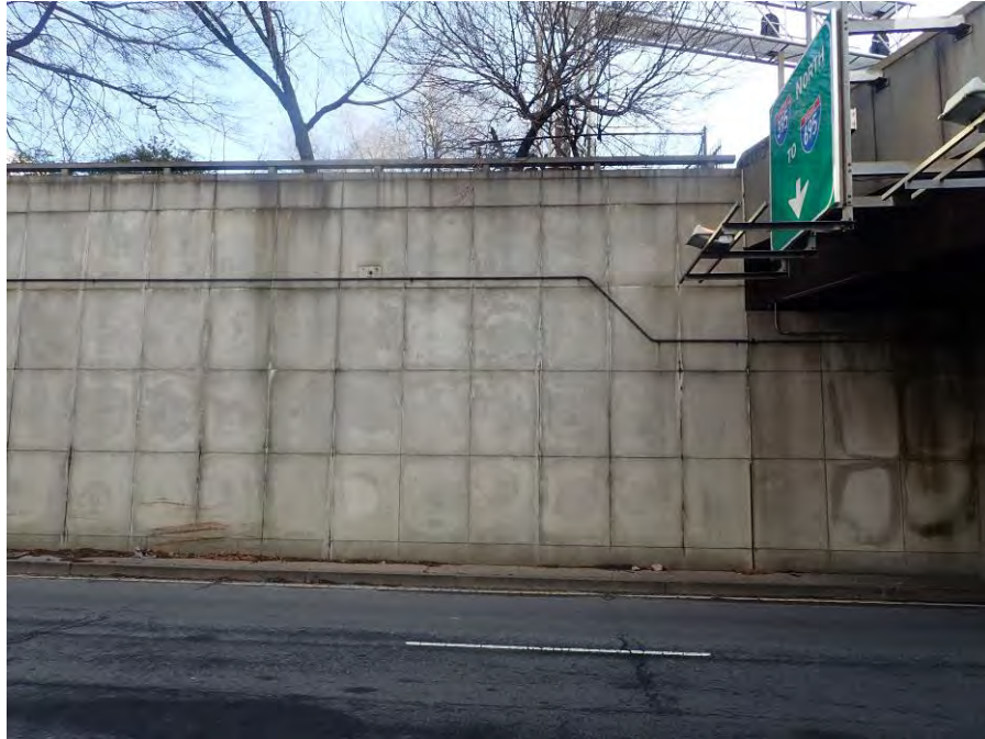
Photograph No. 13 – General View of the Northeast Wingwall
