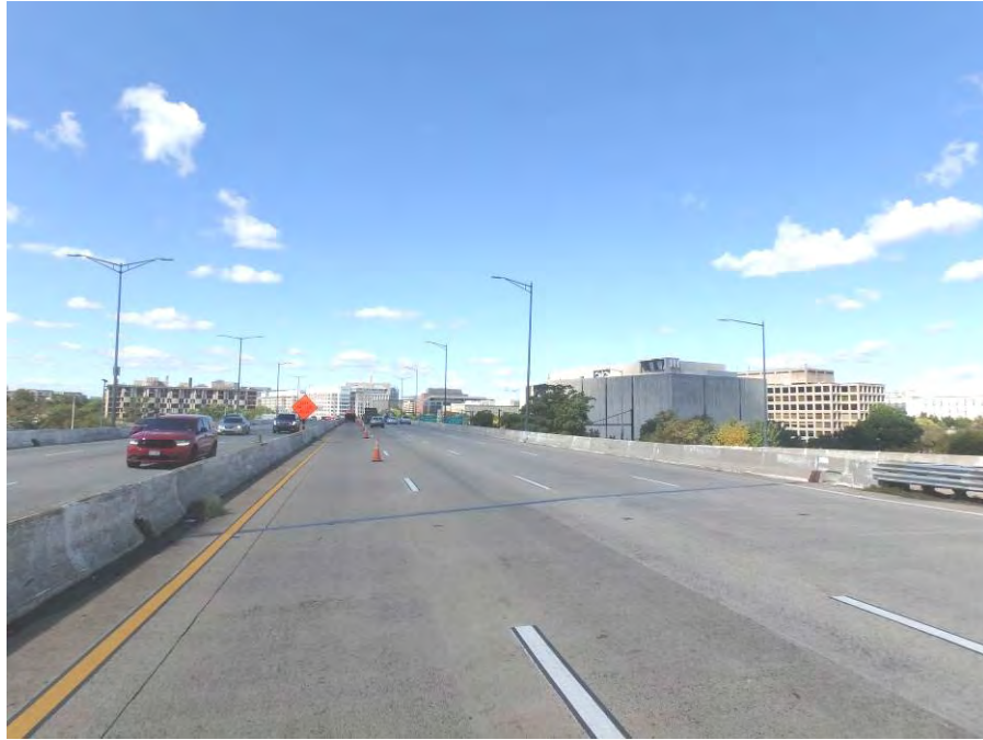
Photograph No. 3 – Westbound Lanes, West Approach, Looking Northwest
