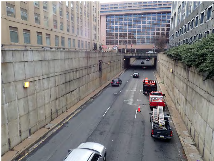
Photograph No. 4 – Looking South from the Top of the Bridge
