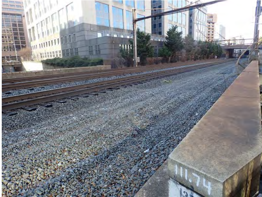
Photograph No. 5 – General View on Top of the Bridge, Looking Southwest
