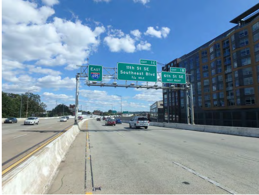
Photograph No. 77 – Overhead Sign Structure for Eastbound Traffic in Span 10
