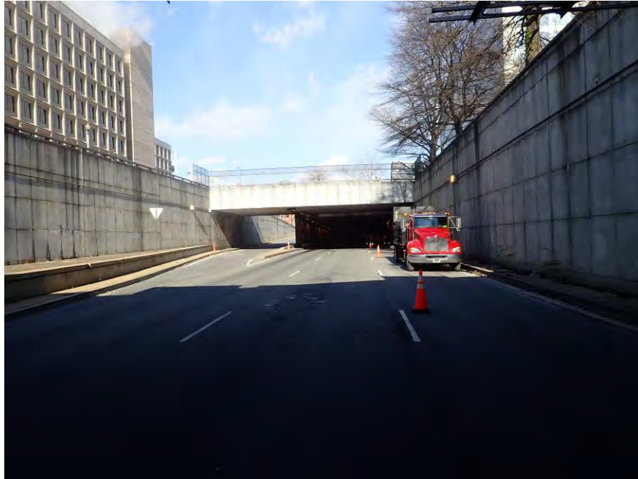
Photograph No. 3 – Looking North from Under the Bridge
