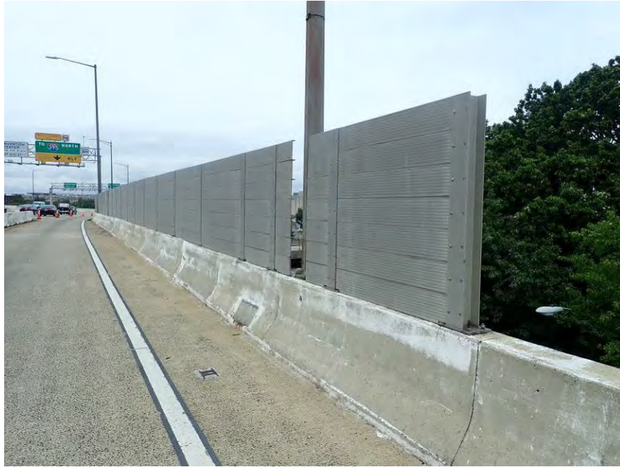
Photograph No. 25 – Typical Protective Railroad Screening (North Parapet of Westbound Lanes Shown, Looking Northwest)
