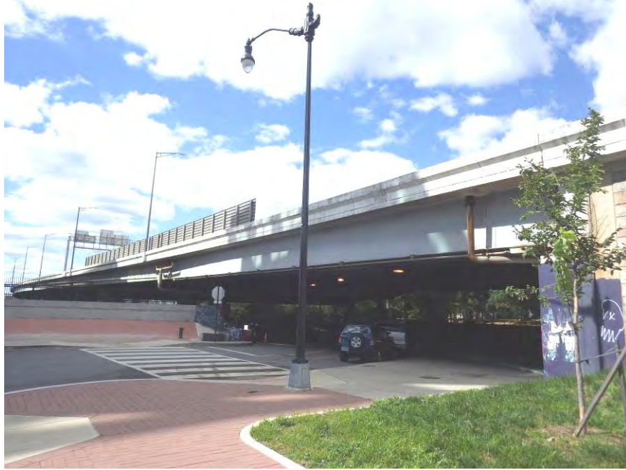
Photograph No. 1 – Partial South Elevation, Looking Northwest at Spans 9 through 12
