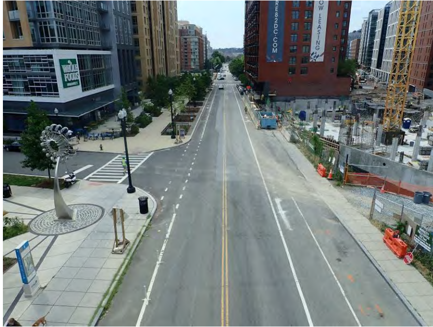
Photograph No. 11 – Looking South from the Top of the Bridge over New Jersey Avenue
