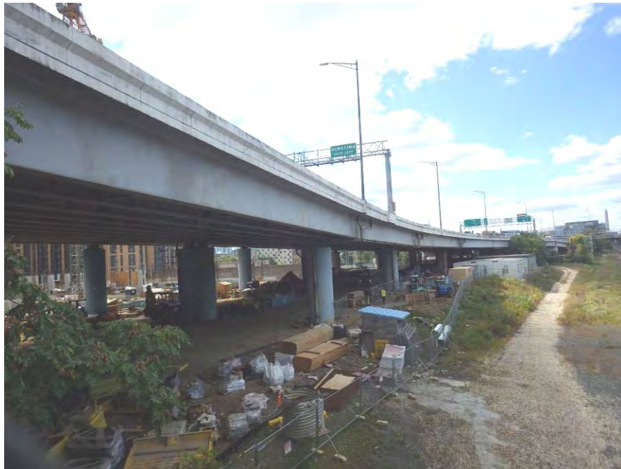
Photograph No. 2 – Partial North Elevation, Looking Southwest at Spans 1 through 6
