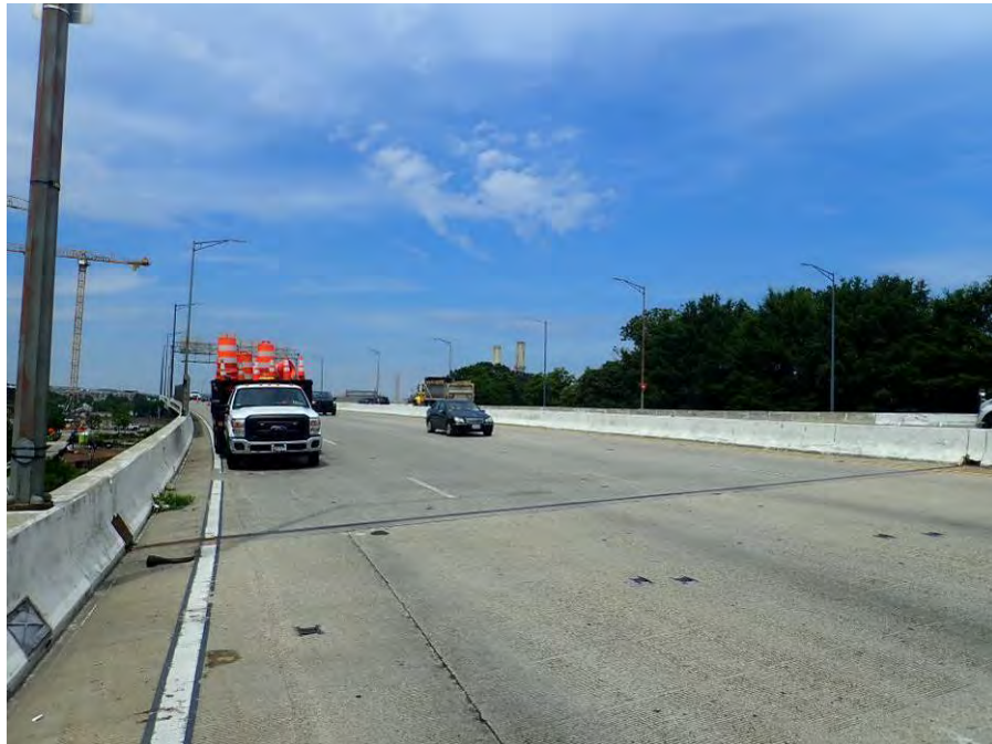
Photograph No. 10 – Eastbound Lanes, East Approach, Looking West
