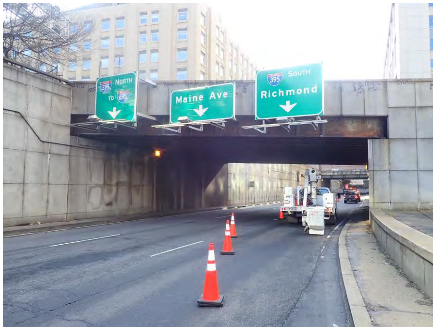
Photograph No. 2 – North Elevation, Looking Southeast
