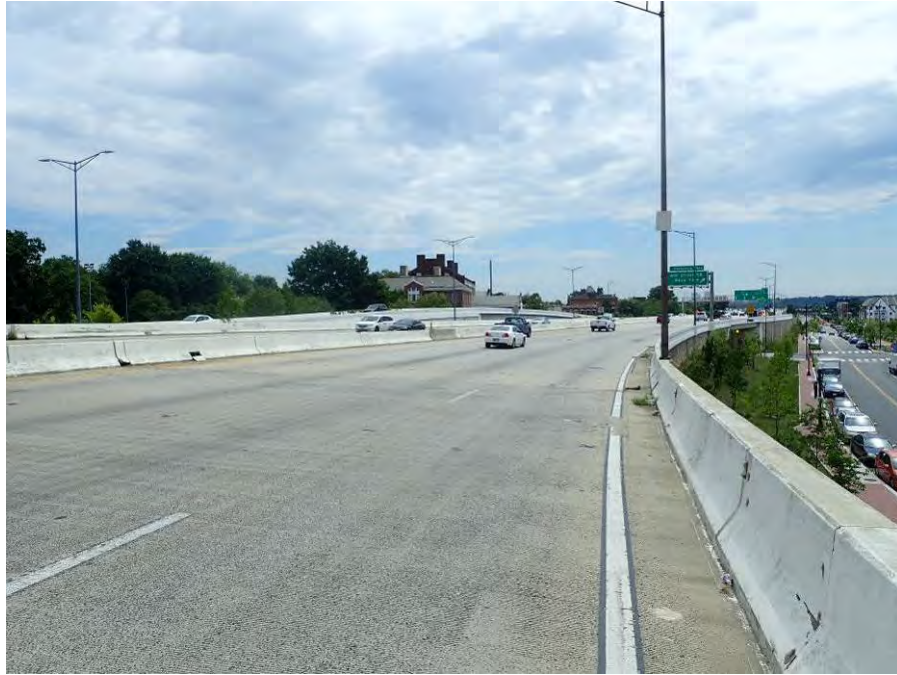
Photograph No. 9 – Eastbound Lanes, East Approach, Looking East
