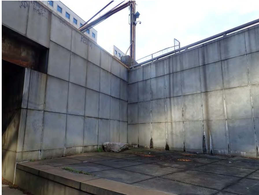
Photograph No. 15 – General View of the Northwest Wingwall
