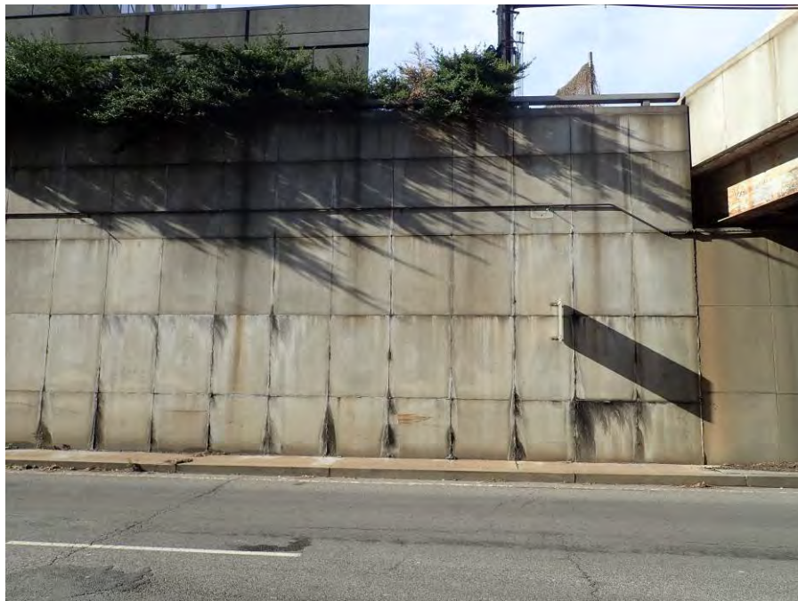
Photograph No. 16 – General View of the Southwest Wingwall
