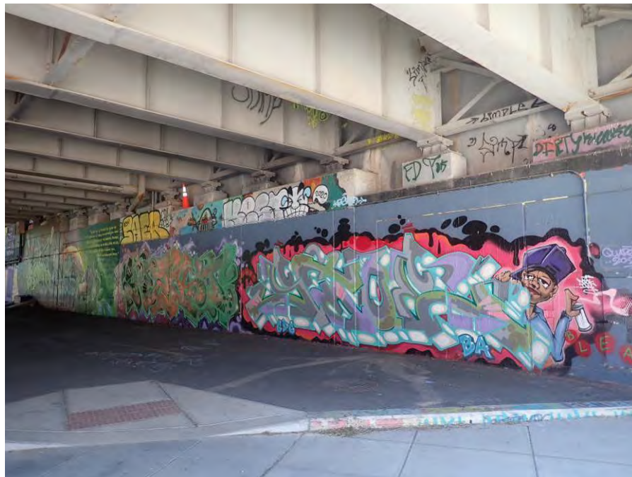
Photograph No. 70 – General View of the East Abutment
