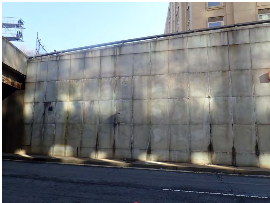
Photograph No. 14 – General View of the Southeast Wingwall
