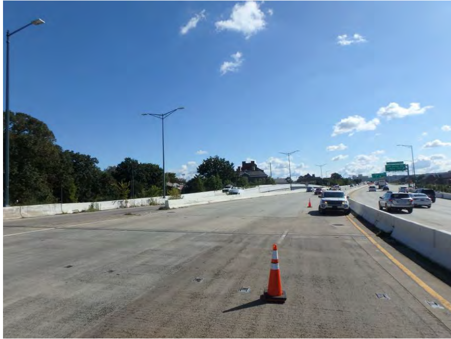
Photograph No. 7 – Westbound Lanes, East Approach, Looking East
