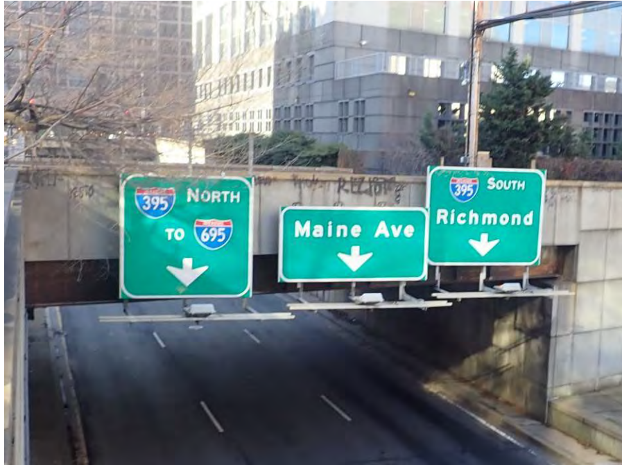
Photograph No. 31 – Traffic Signs on the North Fascia
