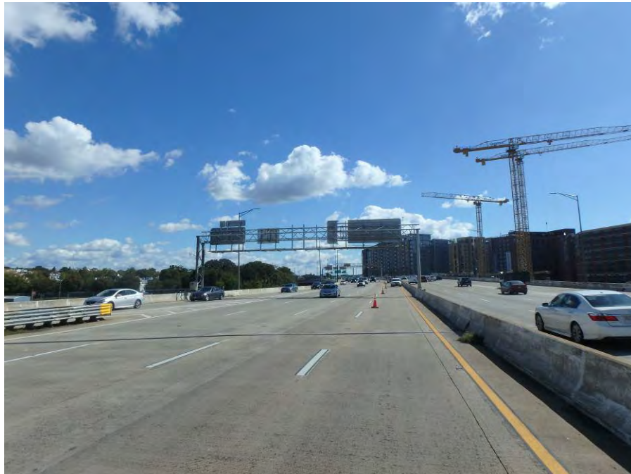
Photograph No. 4 – Westbound Lanes, West Approach, Looking East
