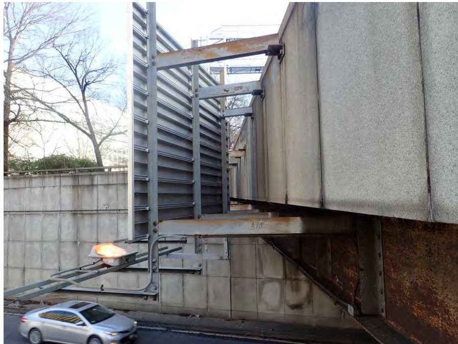
Photograph No. 32 – North Fascia. Note Sign Supports
