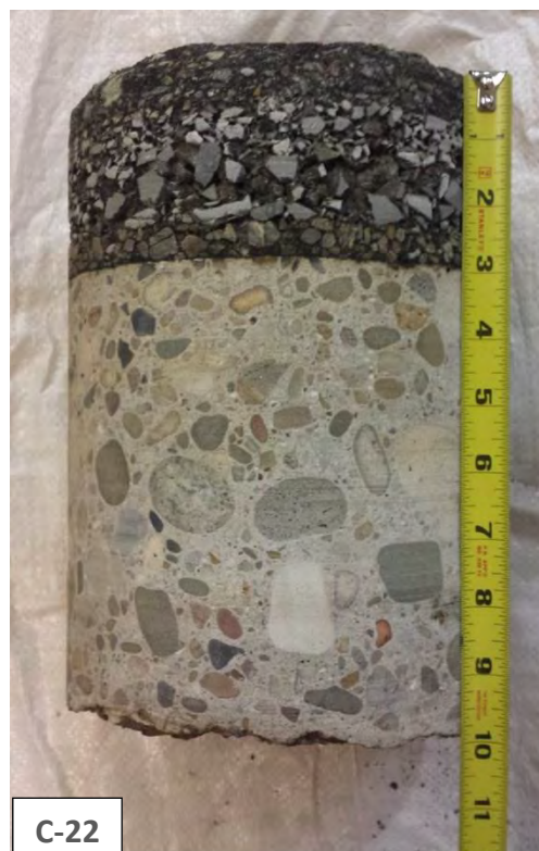
Figure 26-6 | Example of Pavement Core
