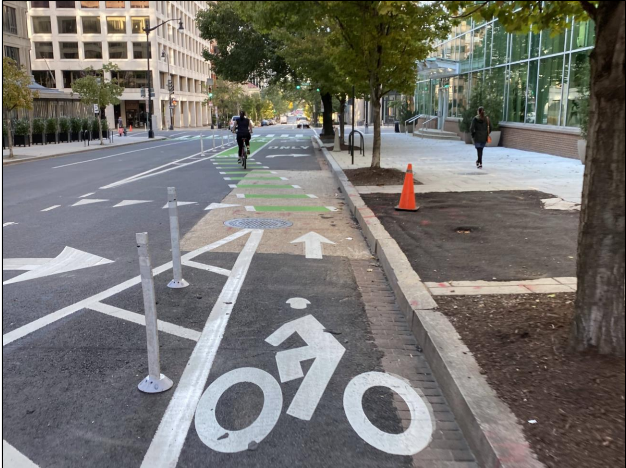
Figure 36 | Dedicated Right Turn Lane and Bicycle Through Lane on M Street NW
