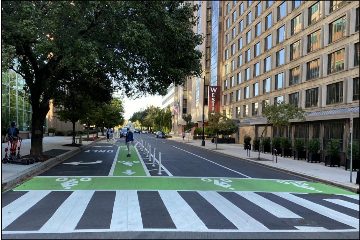
Figure 27 | Intersection Bicycle Box on M Street NW
