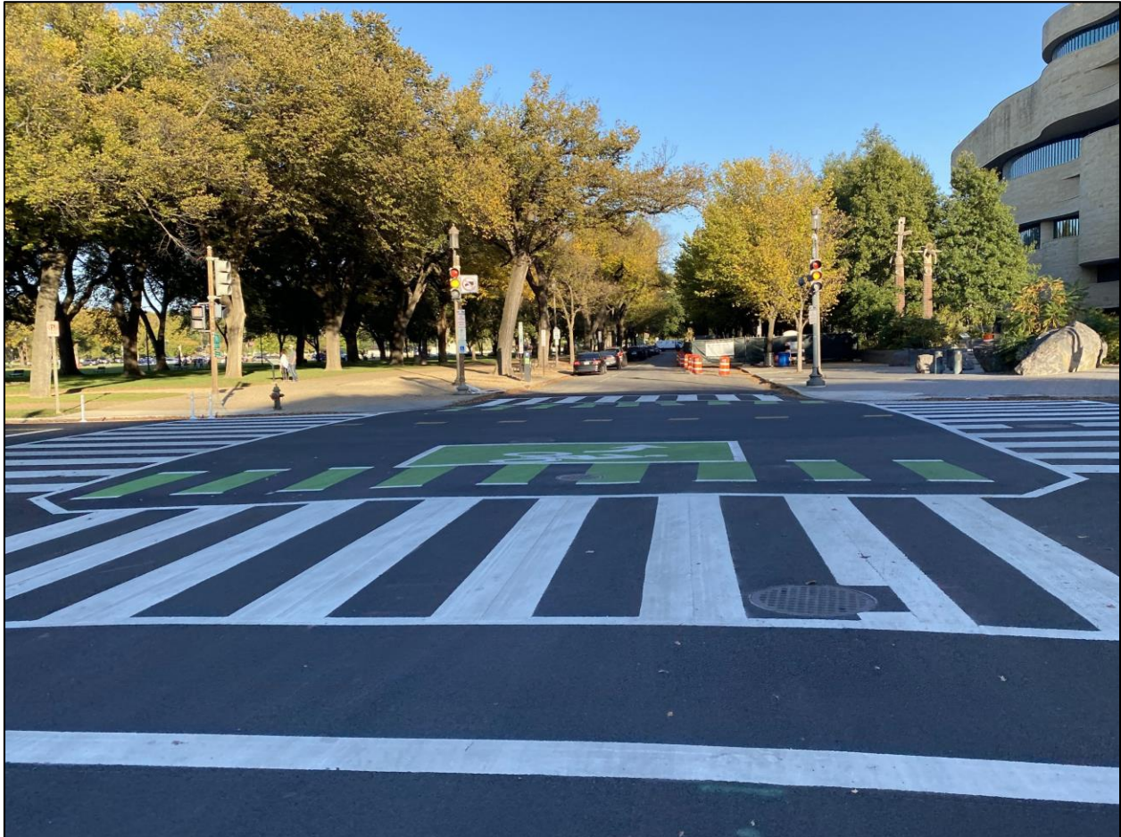
Figure 28 | Two-stage Turn Queue Box on 4 th Street SW at Jefferson Drive SW
