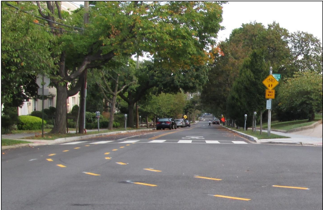
Figure 8 | Shared Lane and Contraflow Bicycle Lane on 42 nd Street NW in Friendship Heights
