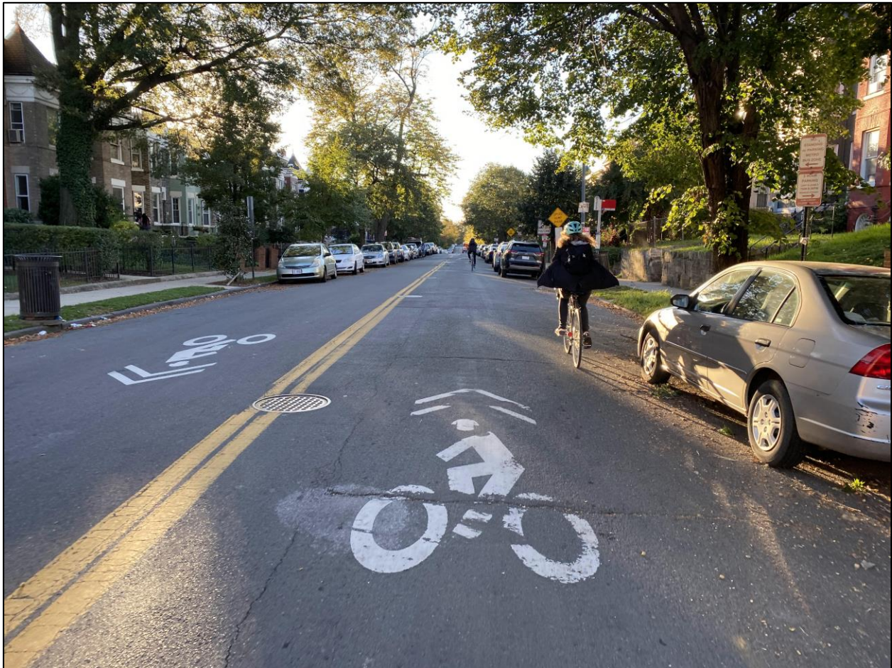
Figure 2 | Shared Lanes on R Street NE
