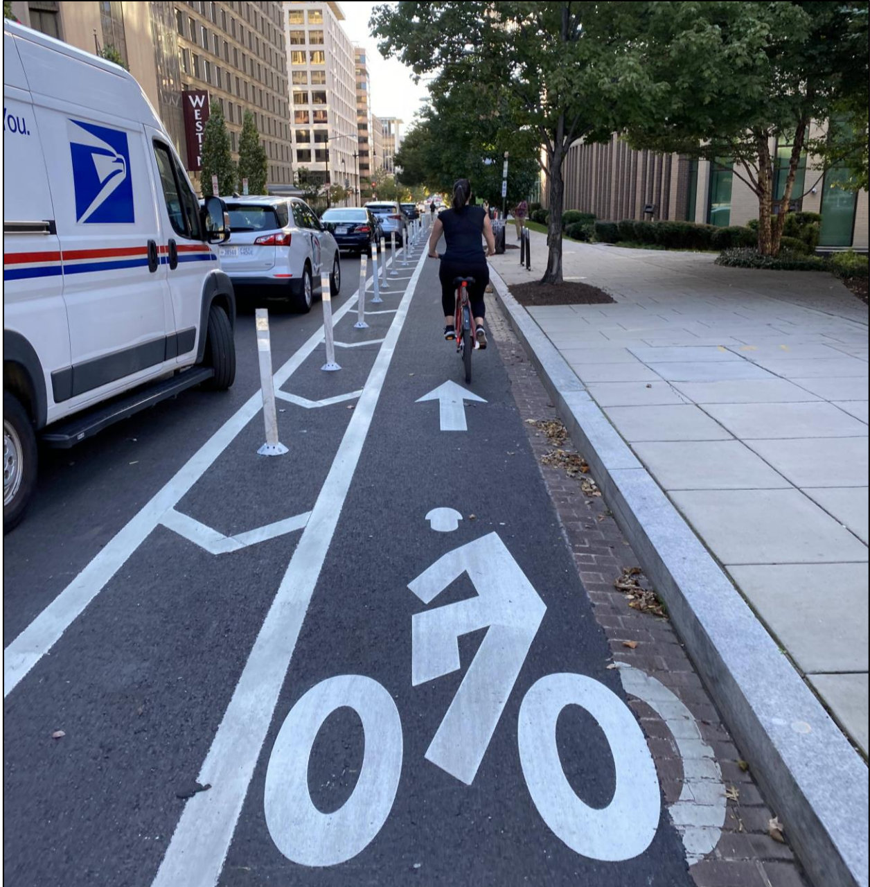
Figure 5 | Protected Bicycle Lane on M Street NW
