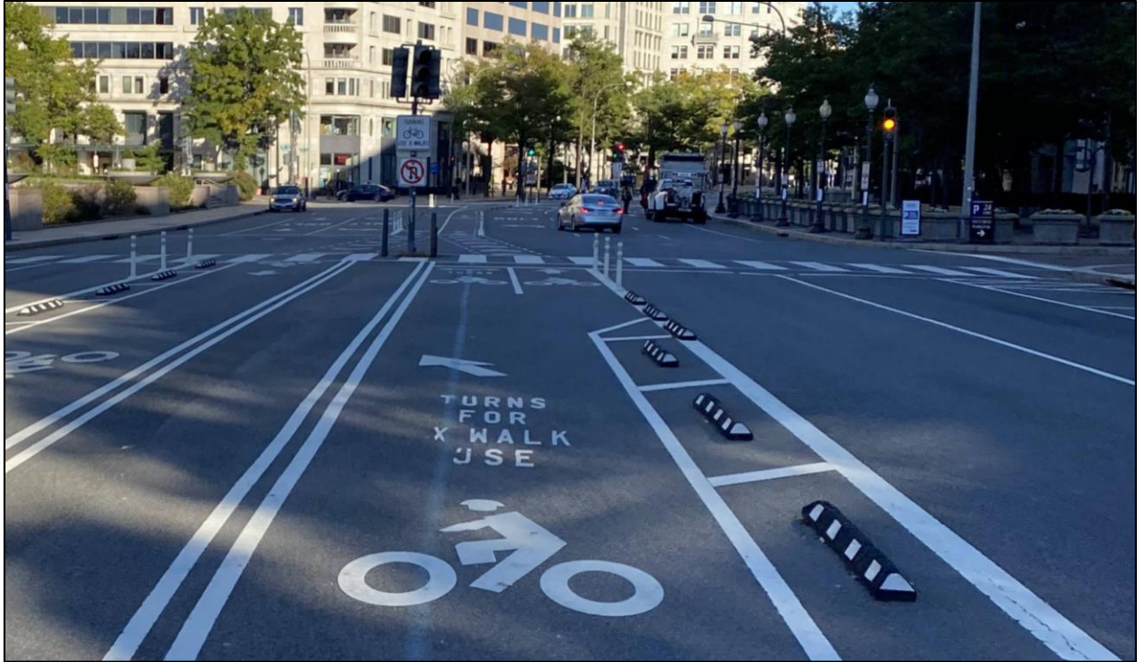
Figure 29 | Bicycle Turn Pocket Approach of Pennsylvania Avenue NW at 13 ½ Street NW
