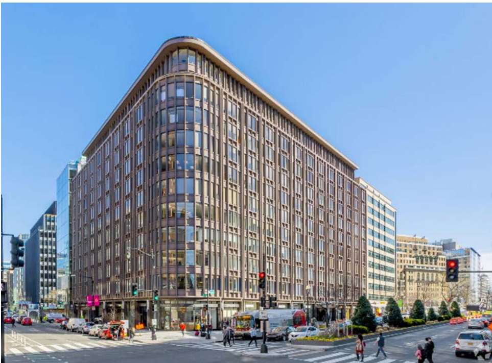
(view from L St NW at Connecticut Ave. NW. Source: Google)
