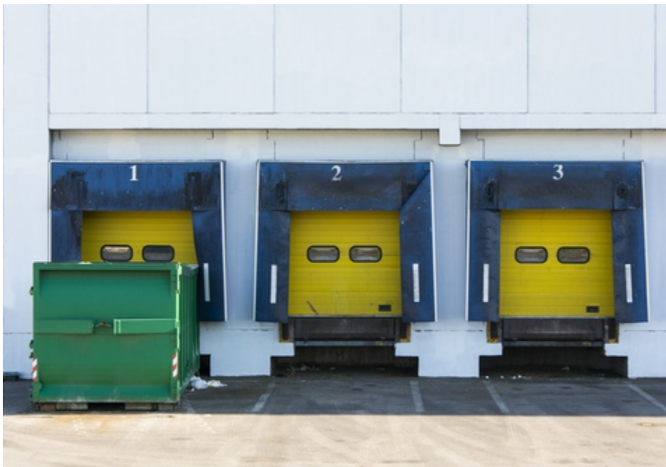
Figure 1-1 | Multiple On-site Loading Berths
