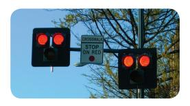
A HAWK (High-Intensity Activated crossWalK) signal is a signal-beacon designed to help pedestrians safely cross busy streets.
