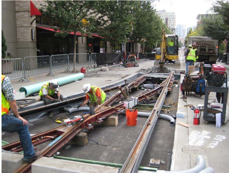
Figure 5-20 | Embedded Track Frog
