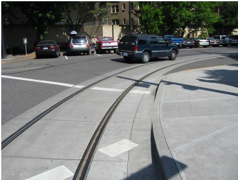
Figure 5-7 | Concrete Slab Track
