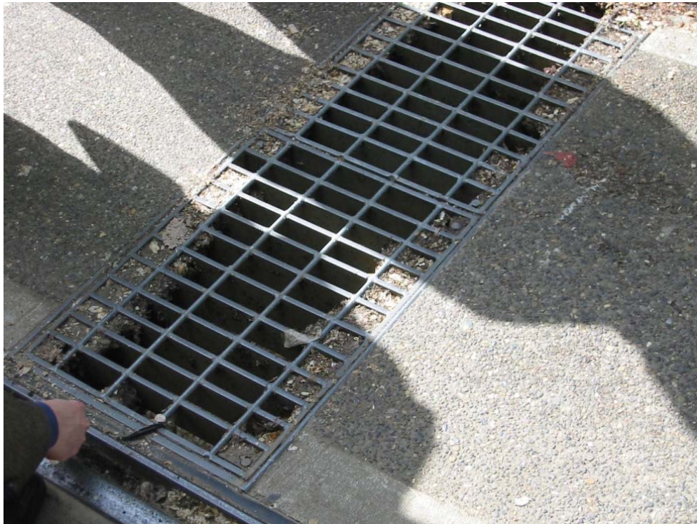
Figure 5-13 | Track Drain Example
