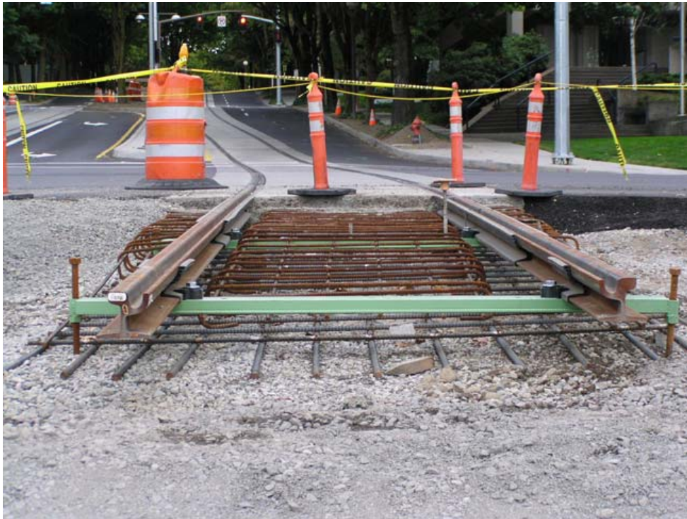
Figure 5-12 | Embedded Track Slab Construction
