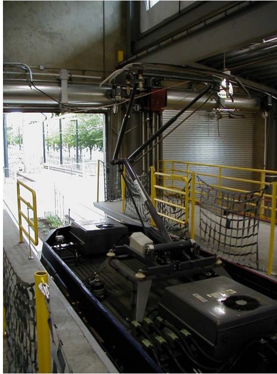
Figure 7-1 | Mezzanine Access to Streetcar Roof
