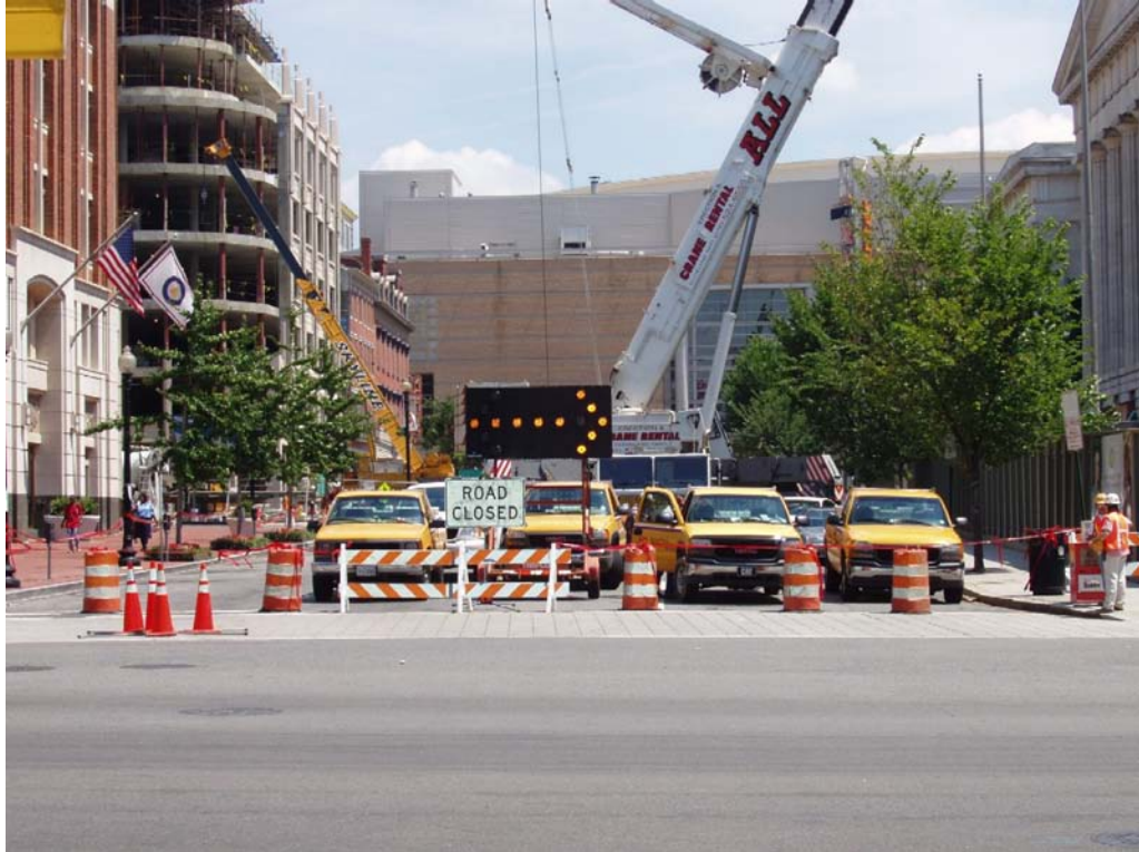
G Street Closure – Crane Operation – 2
