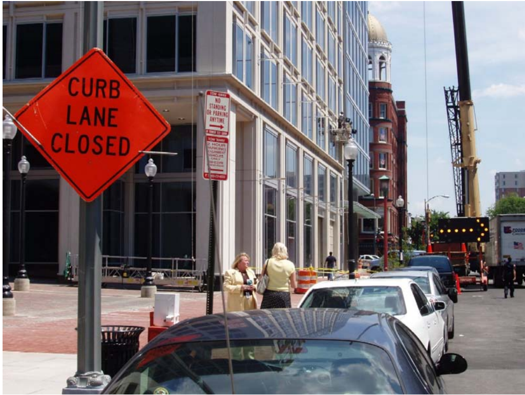
I Street – Partial Closure – Crane Operation – 3
