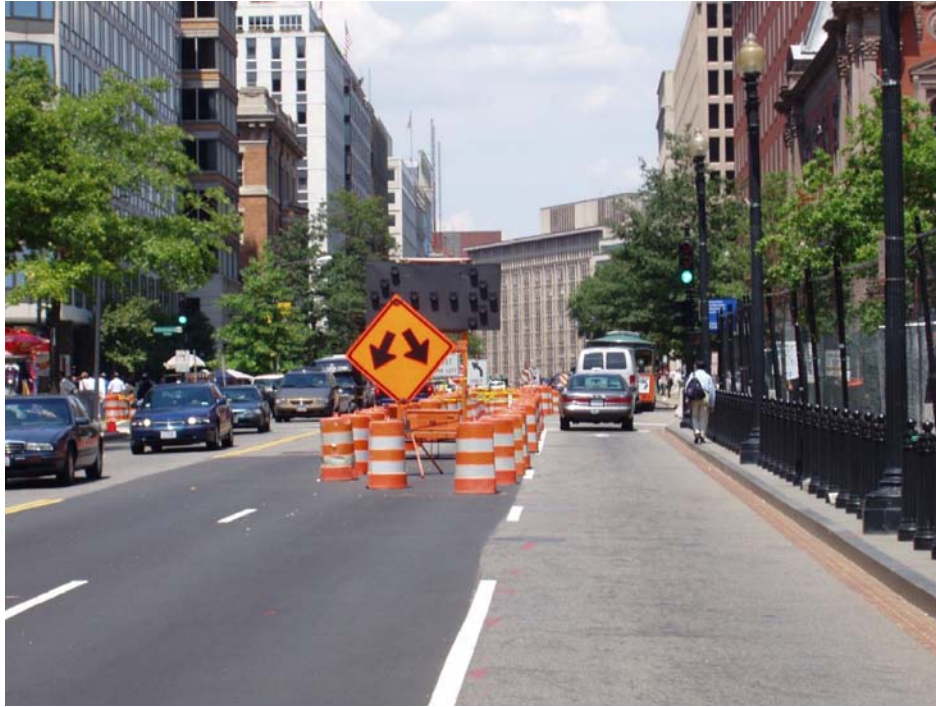
Center Lane Closure
