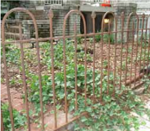
"Wicket" metal fences are commonly found in older sections of the District.
