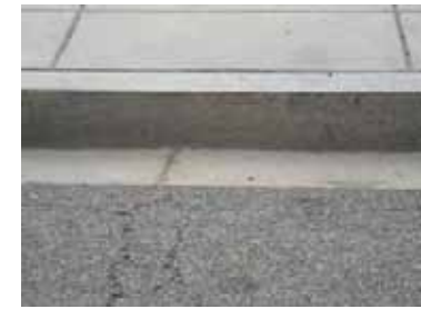
Granite curb with concrete gutter
