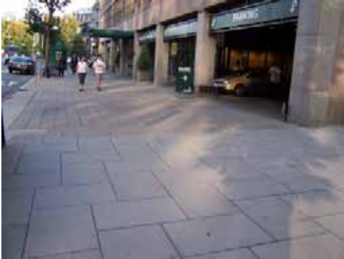
Driveways that cross sidewalks must be flush with the grade of the sidewalk.
