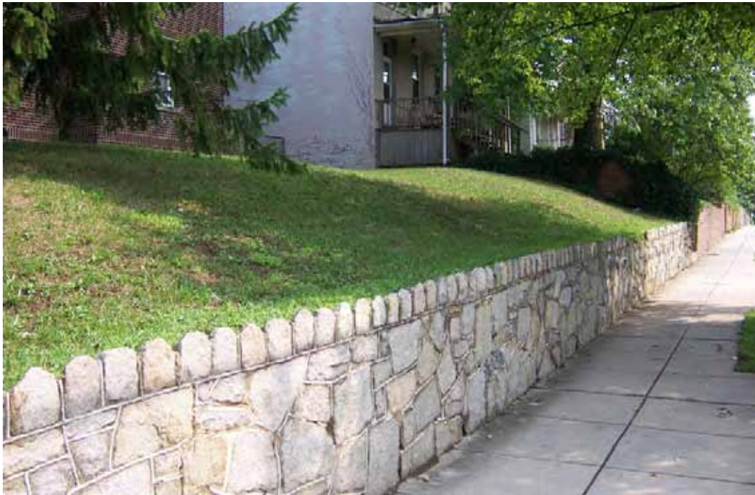
Retaining walls are intended to hold back existing topography.
