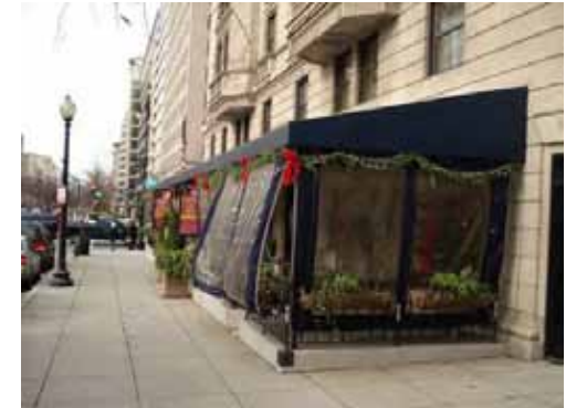
The walls of an enclosed sidewalk café may be solid up to 36 inches from the sidewalk, but the remaining wall must be a transparent material.
