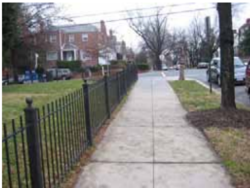
The standard paving for sidewalks in residential areas is concrete
