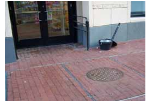
Vaults located in the pedestrian pathway should have solid covers that match the adjacent sidewalk.
