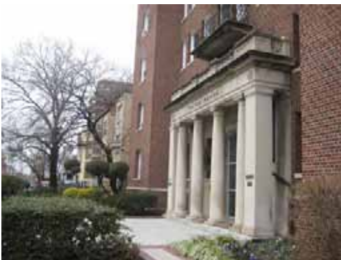
Colonnades may define building entrances but are limited to projecting 6 feet into public space.
