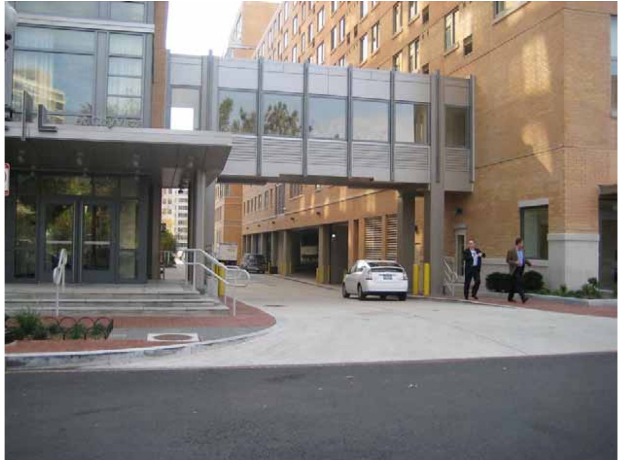
The curb radius for the entrance to a new alley is 10 feet.
