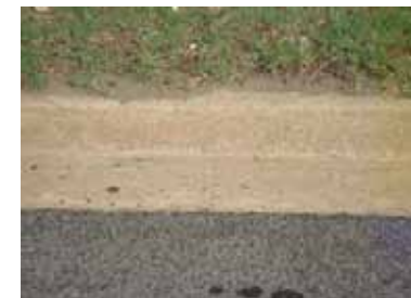
Concrete curb with concrete gutter
