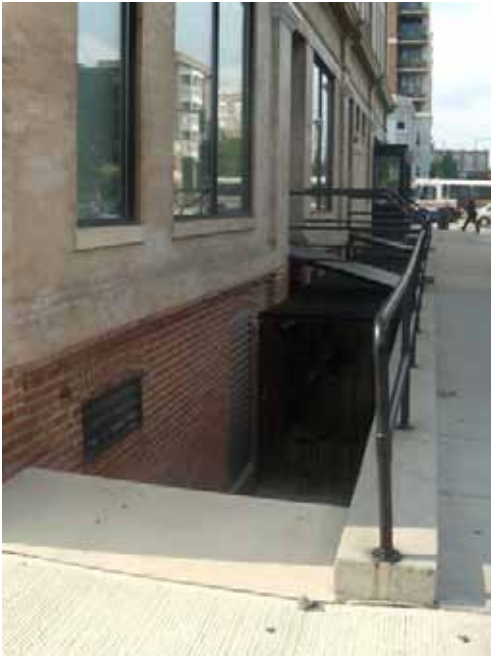
Areaways may be used for lead walks to lower levels, including steps.
