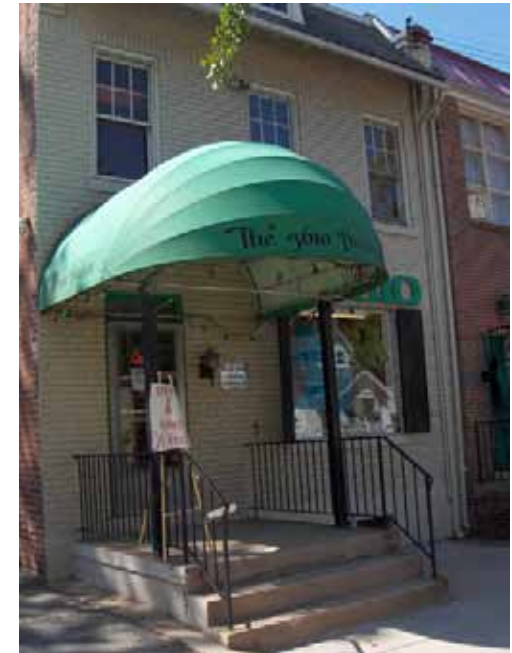
Awnings are temporary roof-like structures attached to buildings, typically over doors and windows.
