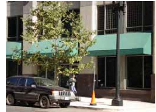
Awnings help to break up the monolithic appearance of large buildings.
