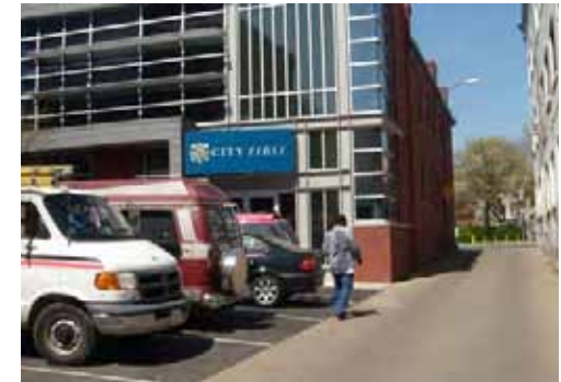
Whenever possible, access to off-street parking should be provided from an alley.
