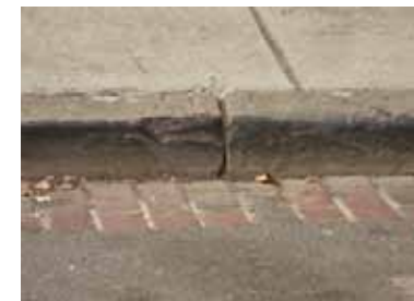
Bluestone curb with brick gutter
