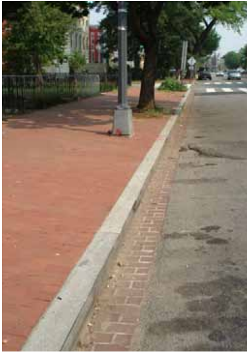
Curbs and gutters define the boundary between the roadway and the sidewalk.
