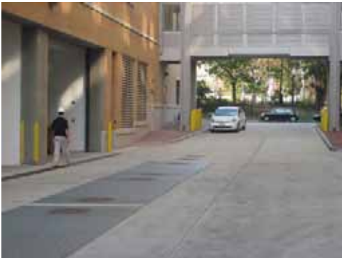
Grated vaults should be located on private property and not in public space.
