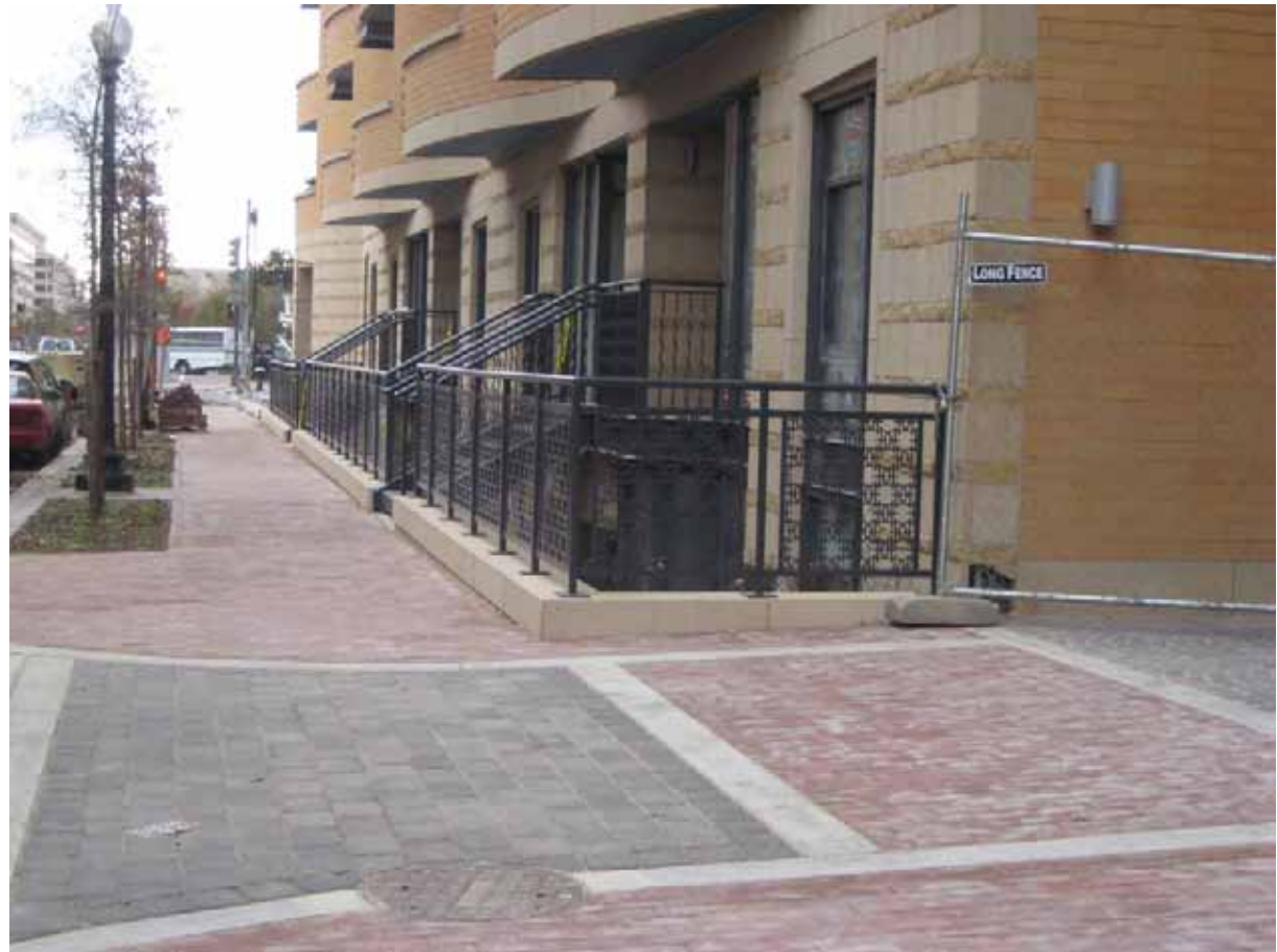
The width of an areaway varies depending on the width of the street and zoning, but all areaways must be protected by a metal railing.
