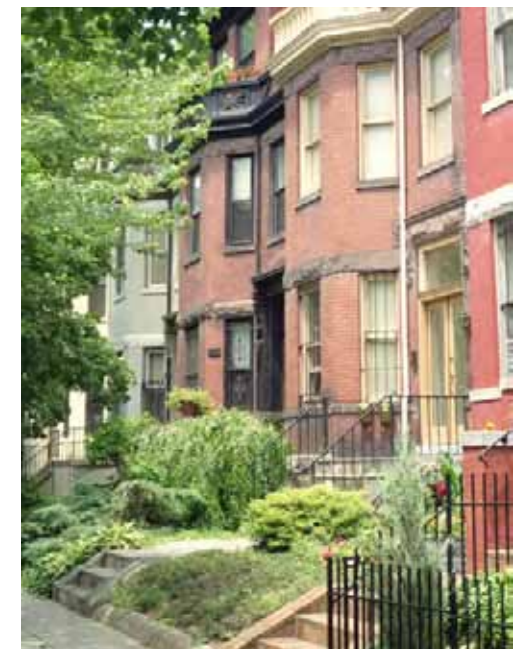
Bay windows promote healthy living by allowing more air and light into building interiors.
