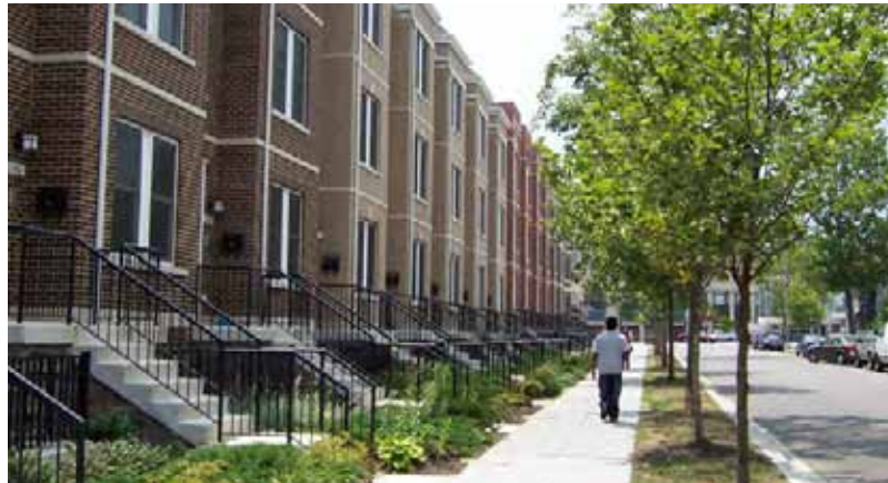
Steps may project into public space as much as 10 feet depending on site conditions.
