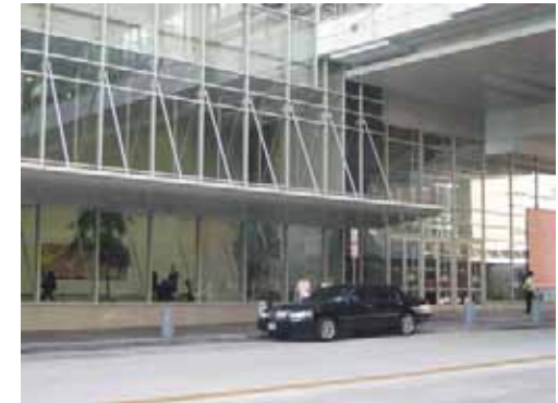
Marquee and canopies that extend along building facades are typically used on buildings that are large gathering places like the convention center.
