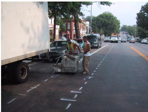
DDOT street maintenance crew applies thermoplastic bike lanes.
