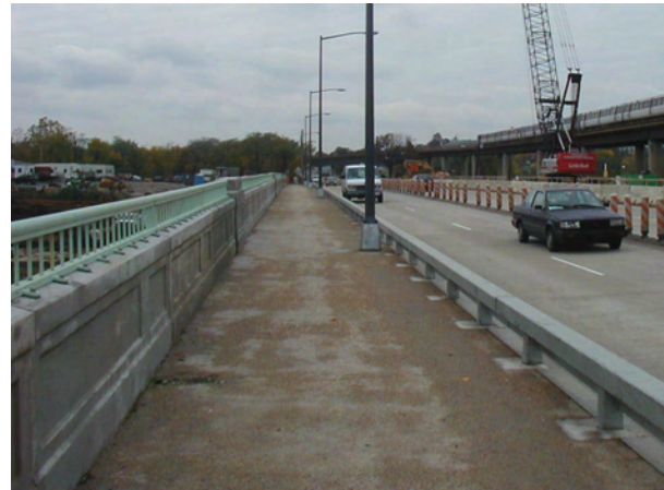
The Benning Road Bridge was improved with wider sidewalks for bicyclists and pedestrians.
