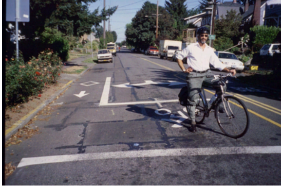
Bicycle Box at an intersection
