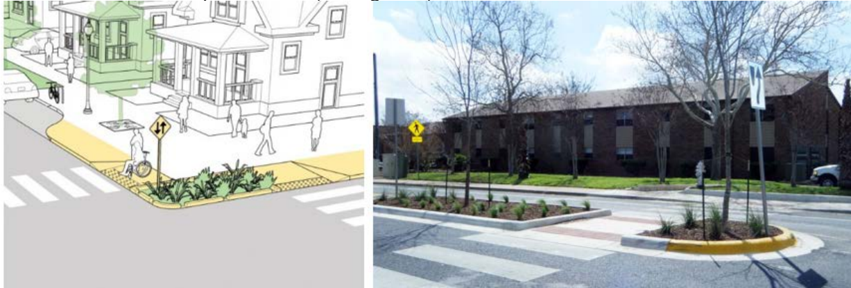
Figure 1: Examples of curb extensions (left, source: NACTO.org) and a median refuge (right, source: NACTO.org);
