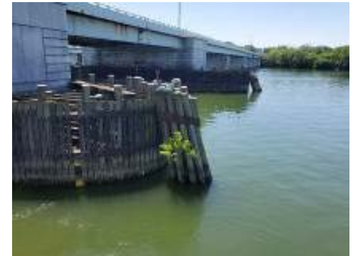
NB I-395 over Potomac: fender system (Arland D. Williams Bridge)
