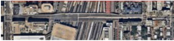
H Street Bridge NE
