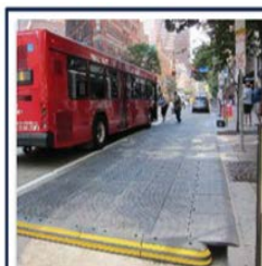
Bulb-outs to allow buses to board from the travel lane and provide more space for passengers to wait
