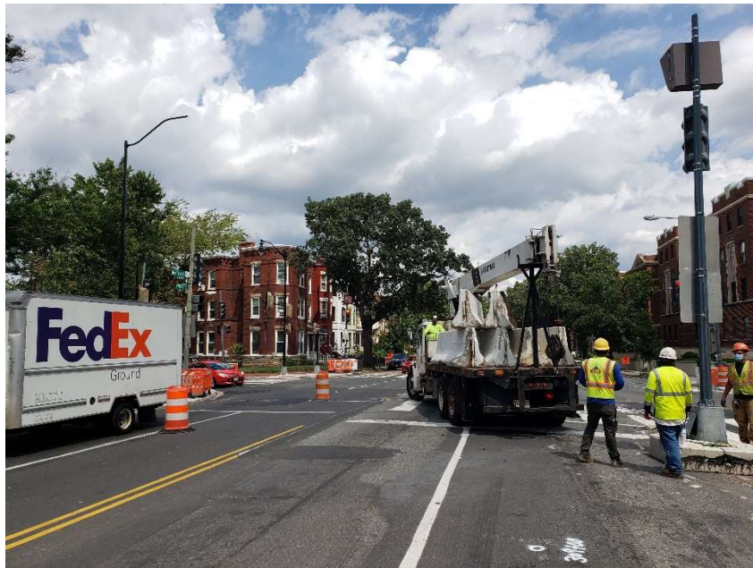
Picture No. 2: 08/17/2020 – Temporary barriers being moved along NY Ave between 1 st St. and NJ Ave. for Phase 4 switch (East View)
