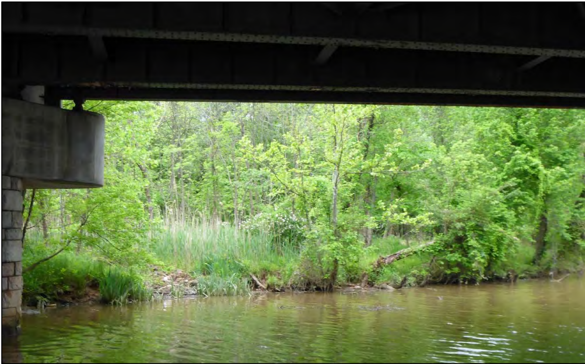
Photograph 17: View of Northwest Embankment, Looking Northwest
