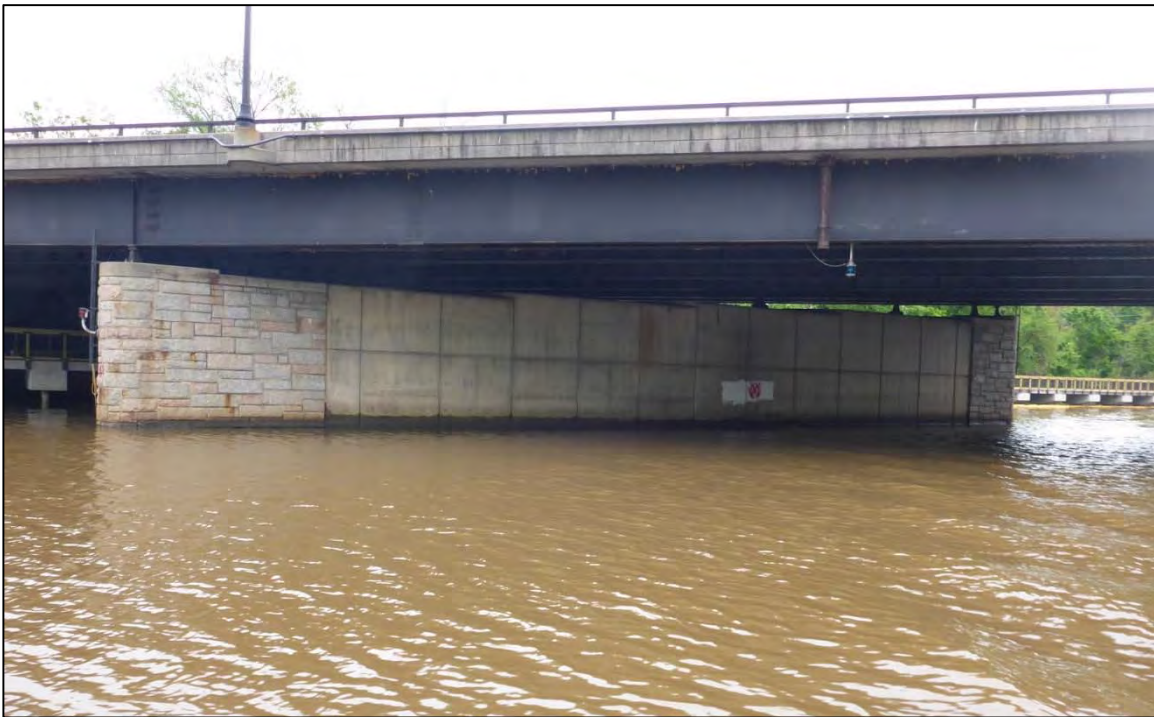
Photograph 10: View of Pier 3, Looking Southeast
