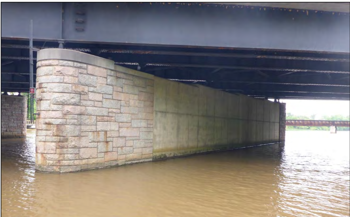
Photograph 4: View of Pier 1, Looking Southeast
