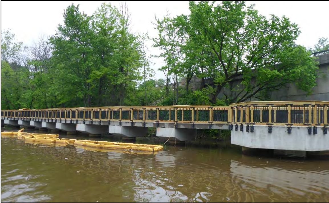
Photograph 19: View of Northeast Embankment and Pedestrian Riverwalk, Looking Southeast
