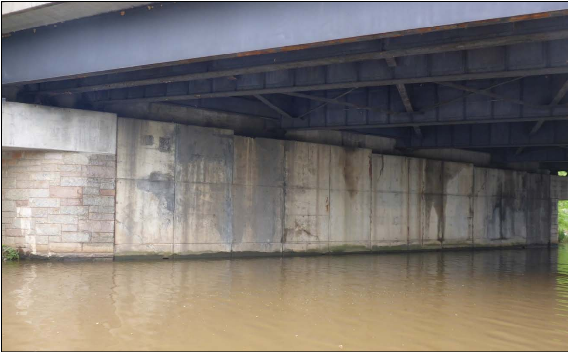
Photograph 3: View of West Abutment, Looking Northwest
