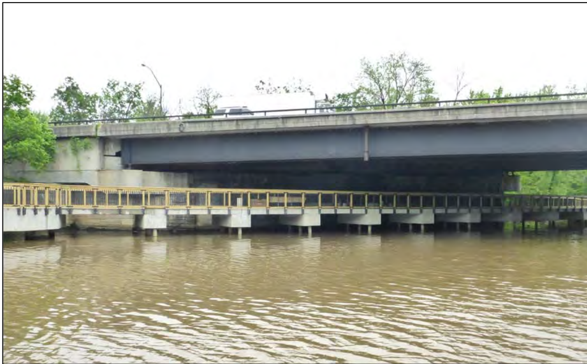
Photograph 14: View of East Abutment and Recently Constructed Pedestrian Riverwalk, Looking Southeast
