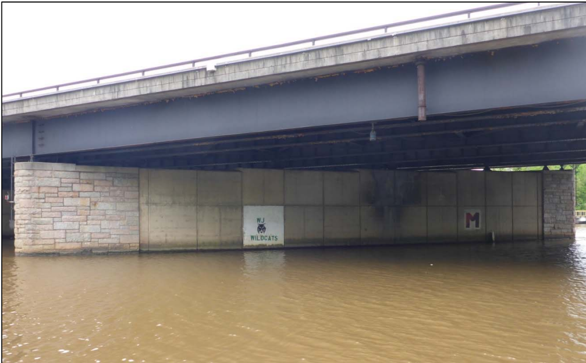
Photograph 7: View of Pier 2, Looking Southeast
