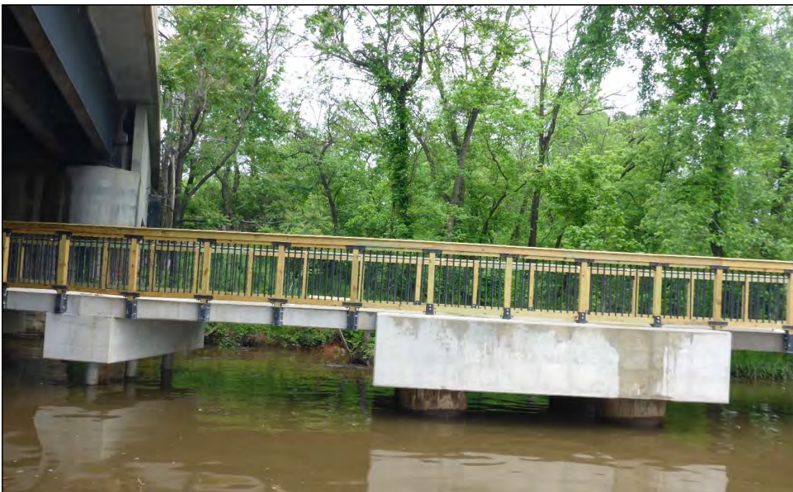
Photograph 18: View of Southeast Embankment and Pedestrian Riverwalk, Looking East
