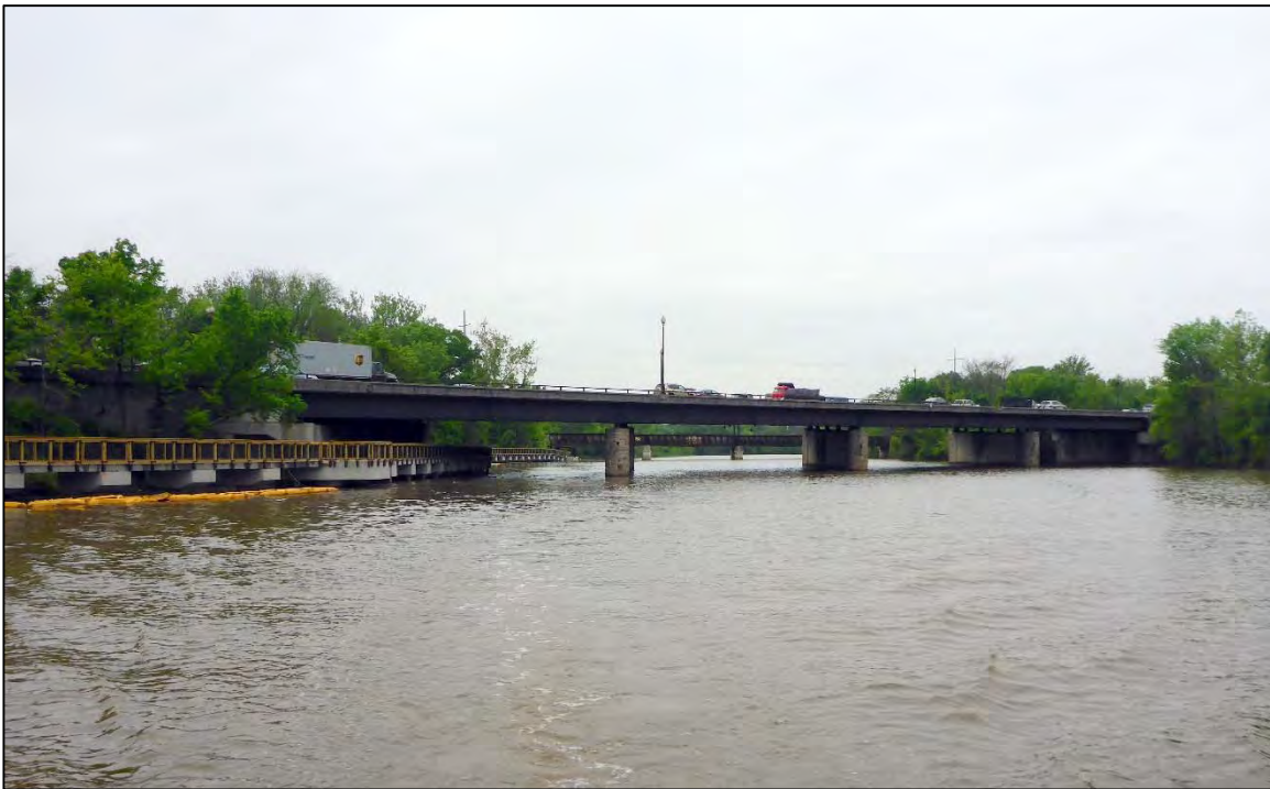
Photograph 2: Overall View of North Elevation, Looking South
