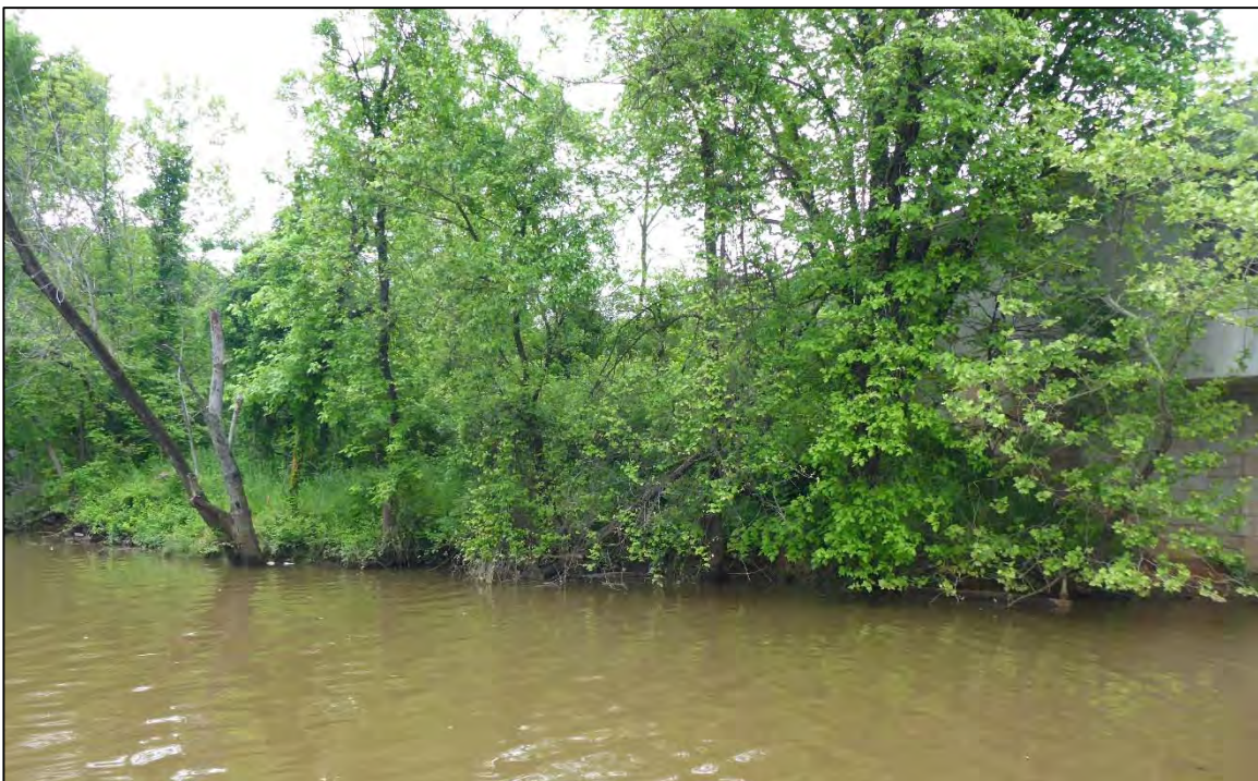
Photograph 16: View of Southwest Embankment, Looking West
