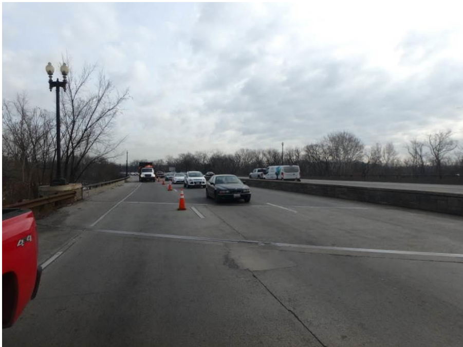
Photograph No. 12 – West Approach, Looking East, Westbound Traffic Lanes
