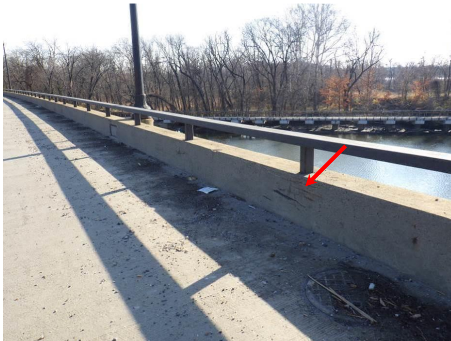
Photograph No. 18 – Typical Reinforced Concrete Parapet with Metal Railing Mounted on Top. Note Minor Scrape Marks (Arrow)
