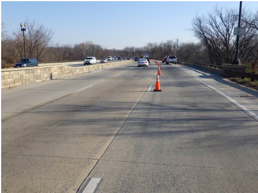
Photograph No. 10 – West Approach, Looking East, Eastbound Traffic Lanes
