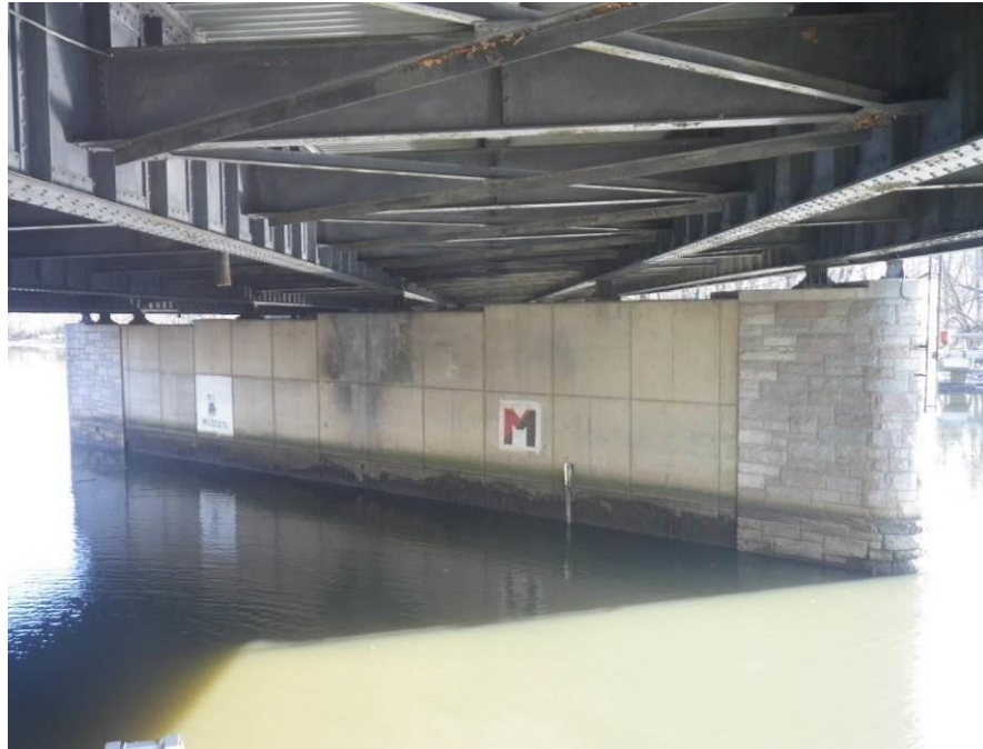
Photograph No. 43 – Pier 2, West Face
