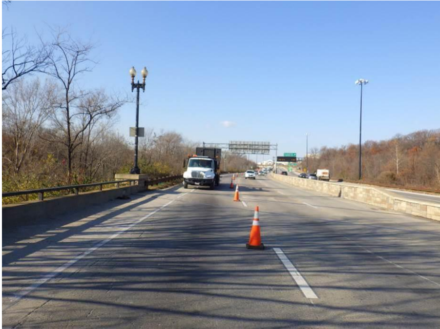
Photograph No. 9 – West Approach, Looking West, Eastbound Traffic Lanes
