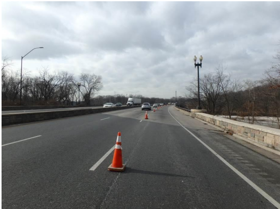
Photograph No. 8 – East Approach, Looking West, Westbound Traffic Lanes
