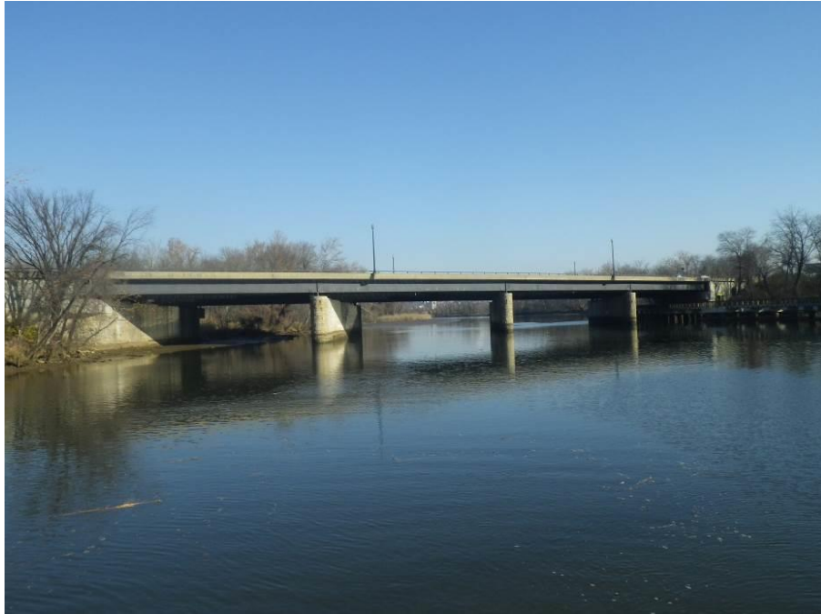
Photograph No. 1 – South Elevation, Looking North
