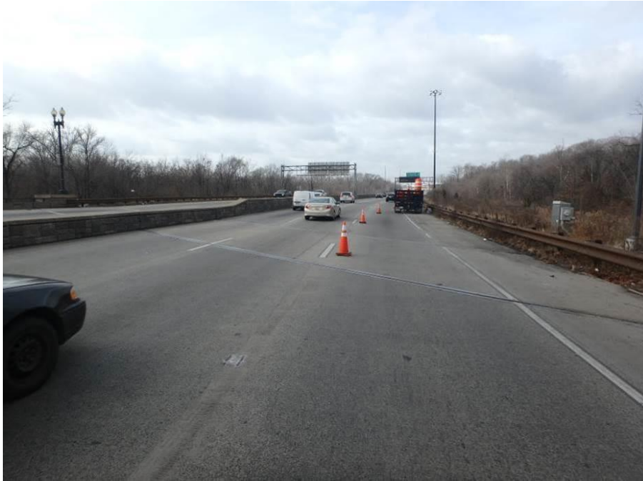
Photograph No. 11 – West Approach, Looking West, Westbound Traffic Lanes
