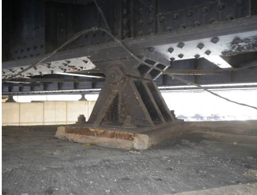
Photograph No. 39 – Typical Fixed Bearing at Pier 2, Bearing 3 Shown, Looking Southeast
