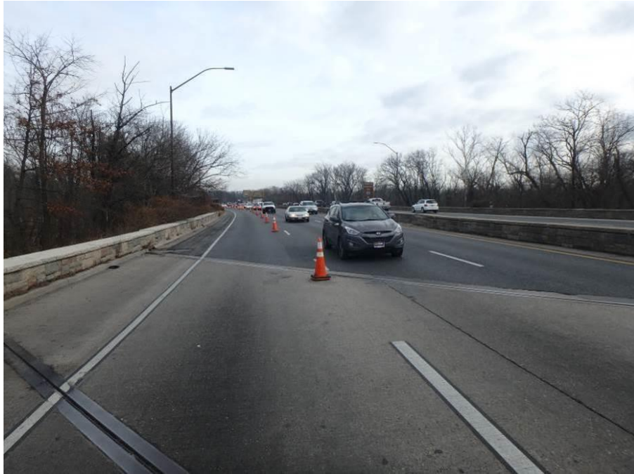
Photograph No. 7 – East Approach, Looking East, Westbound Traffic Lanes
