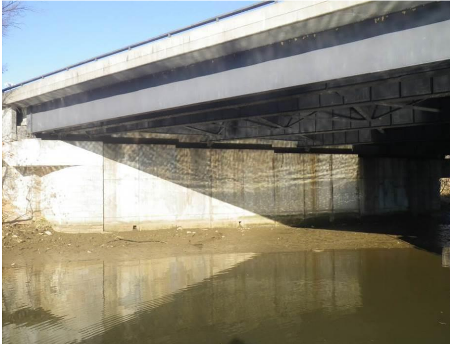
Photograph No. 41 – General View of the West Abutment, Looking Northwest
