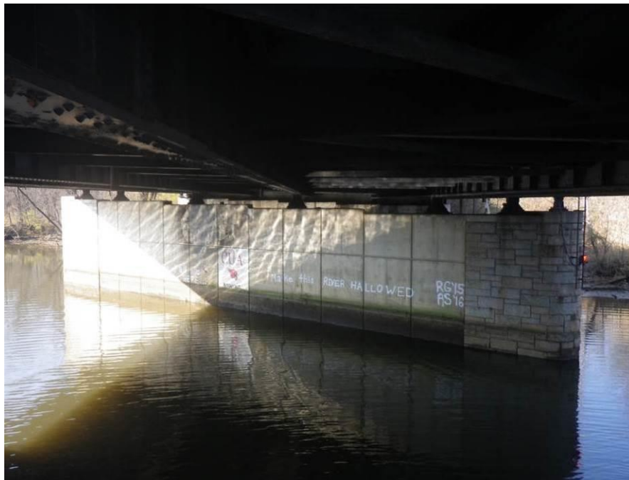
Photograph No. 42 – Pier 1, East Face
