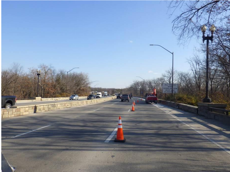
Photograph No. 5 – East Approach, Looking East, Eastbound Traffic Lanes
