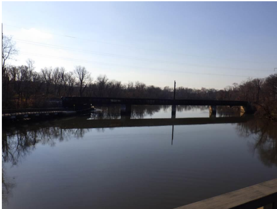
Photograph No. 4 – Looking South from the Top of the Structure
