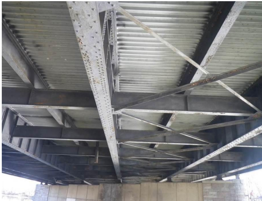
Photograph No. 32 – Girder Span Superstructure, Span 2 Shown, Looking East
