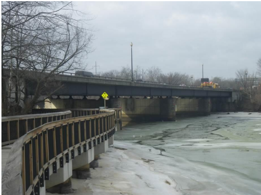
Photograph No. 2 – North Elevation, Looking Southwest
